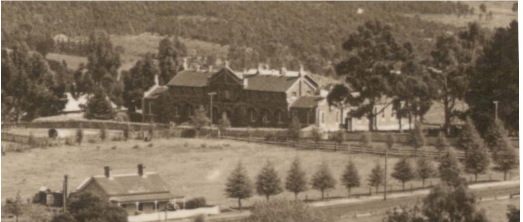
Hospital St. (North of Raglan St. East of Vincent St.) The foundation stone was laid in 1861.
